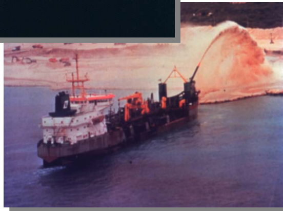
Dredging and Disposal
