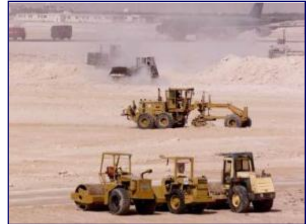
RED HORSE Constructs Aircraft Ramp
